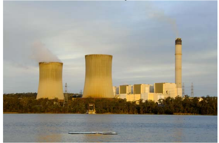
Tarong Power Station
