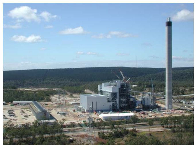
Construction of Tarong North nears completion in 2003
