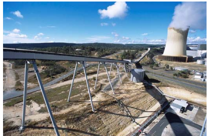
Coal to Tarong North is supplied from the adjacent Meandu Mine via conveyor
