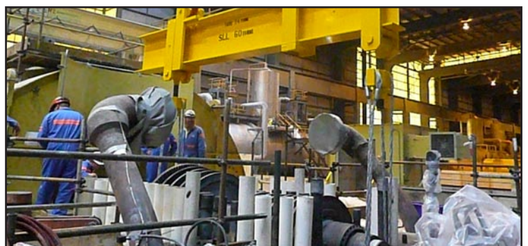
Overhaul of Unit 2 in progress.
